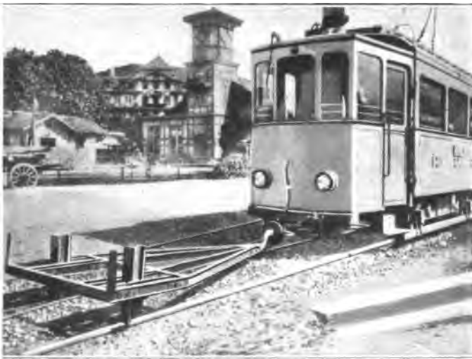
Pushed by the Street Car, This Steel Frame Removes Dirt and Ice from the Tracks. The Steel Uprights, Seen at the Left, can be Adjusted to Fit a Track of Any Gauge
